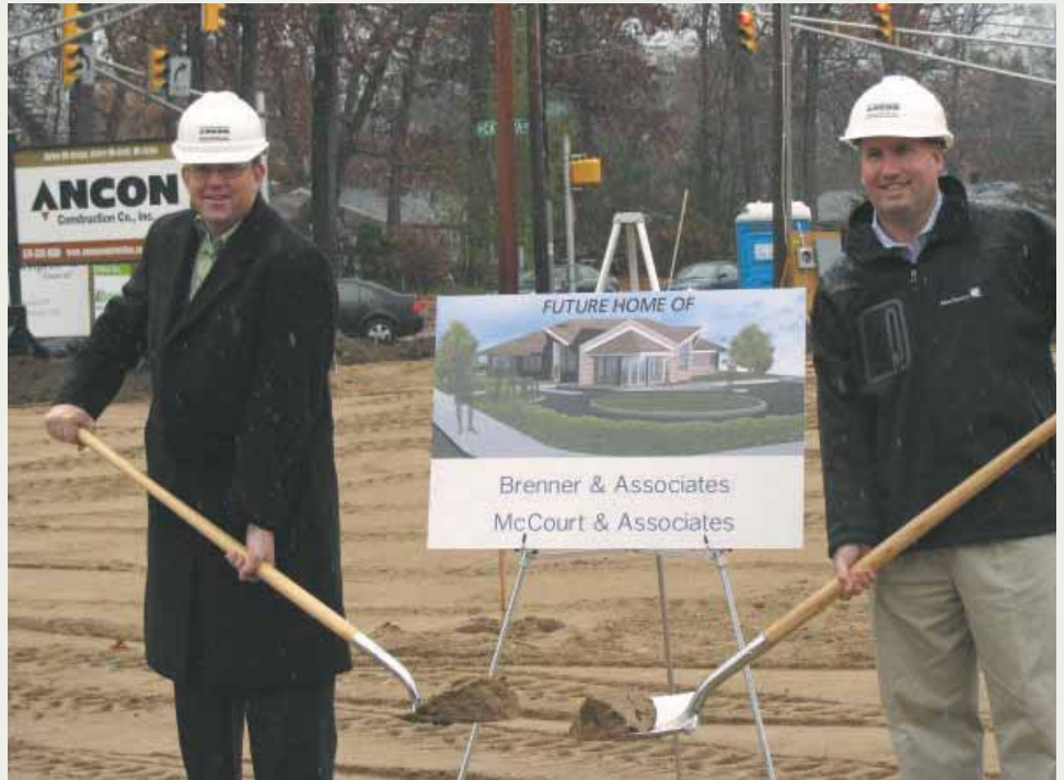
Erik Brenner and Bruce McCourt dig in at the groundbreaking for their new office building.
